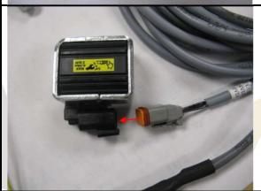
Designated connector on valve harness connects to the float solenoid as shown in photo following installation on Craig valve
